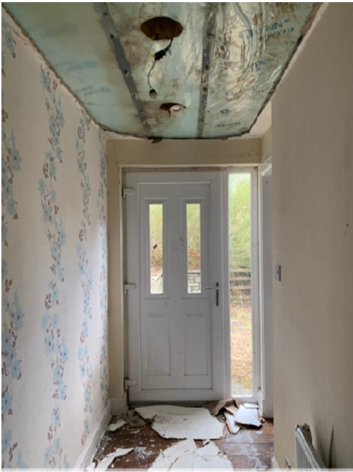
Fig. 3 & 4 - examples of collapsed ceilings and dilapidation in the existing Cottage north-east wing.
