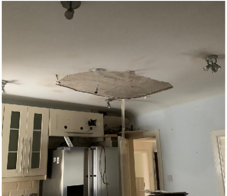
Fig. 3 & 4 - examples of collapsed ceilings and dilapidation in the existing Cottage north-east wing.
