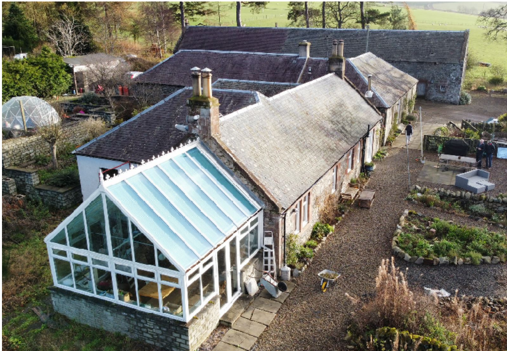
Fig 8 - view of Ratchill looking east, showing the tightly-knit building group.
