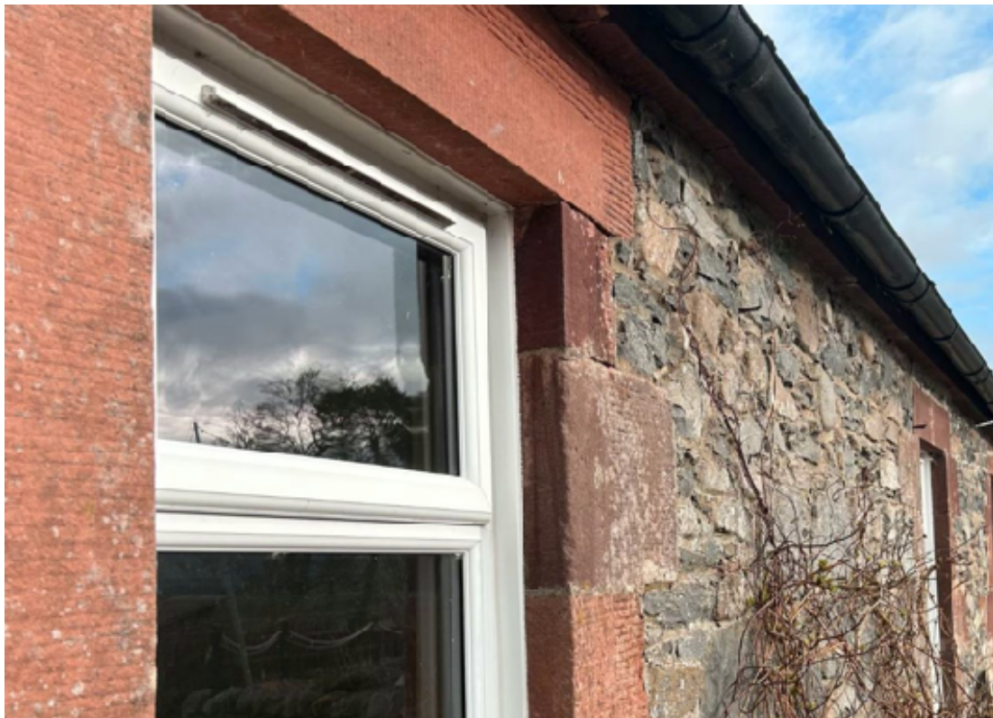
Fig 22 - Existing uPVC windows on Cottage in non-traditional style
